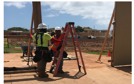
Construction site in April 2018 Photo by Keona Blanks
